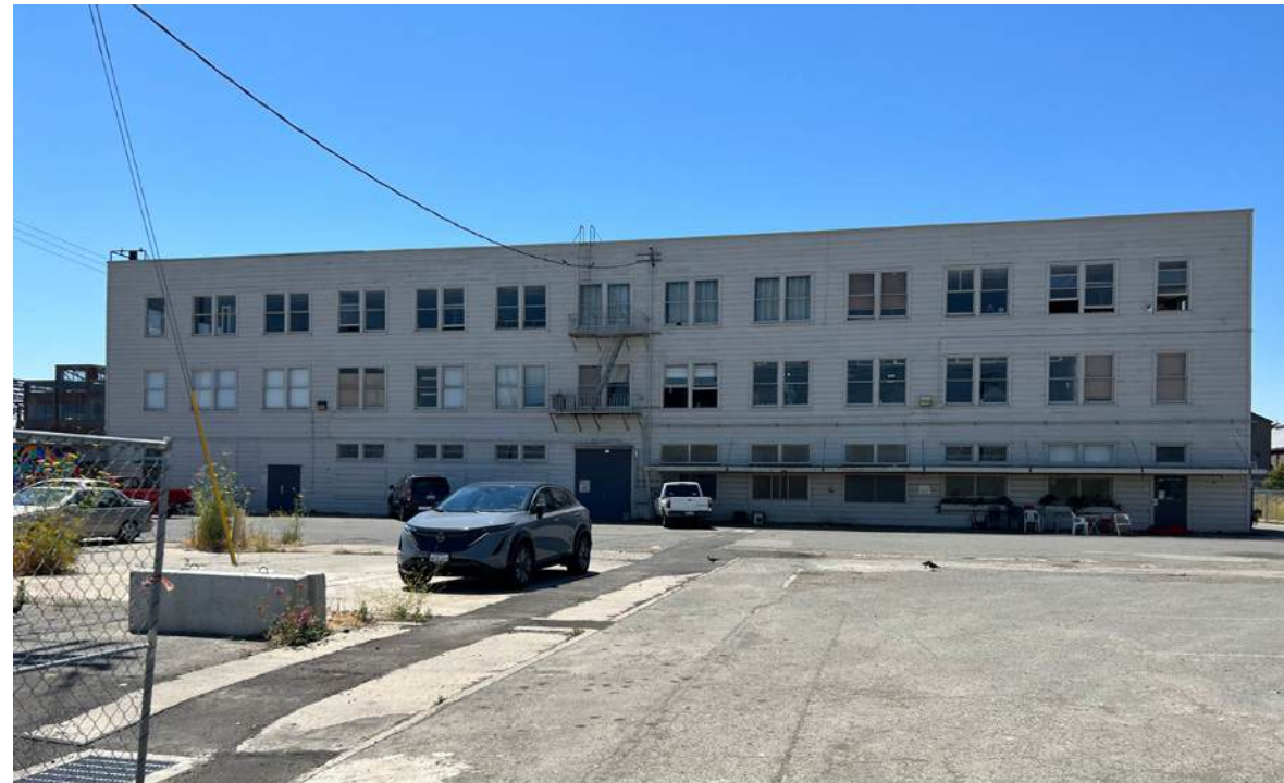
Exterior view of the existing Noonan Building
